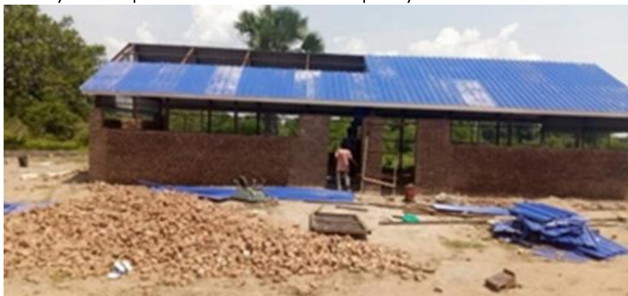
Figure#2 Image1: Anyienyagal Primary School during renovation process
