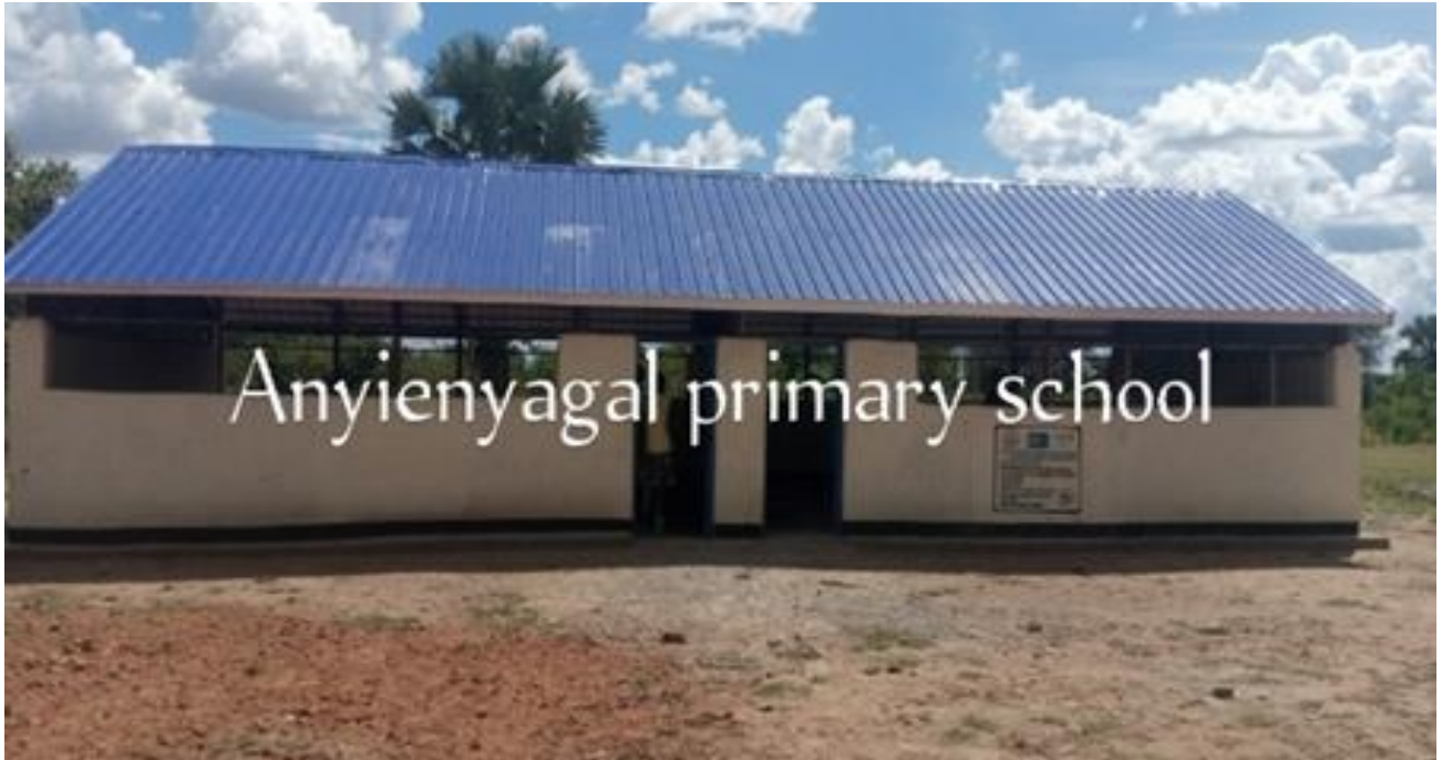
Image2: Anyienyagal Primary School after renovation
