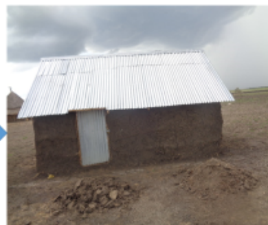
After completion of the construction.
