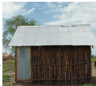
After construction of new structure
