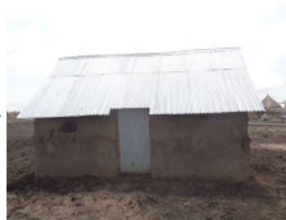
Kuetrengke After construction.
