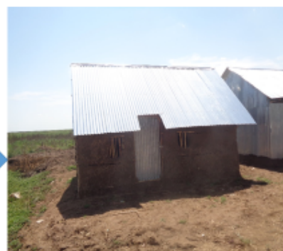
The new Maker OTP structure constructed within the premises of the health facility.
