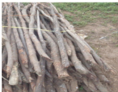
Local poles brought by community to the site mobilized by the local authorities.
