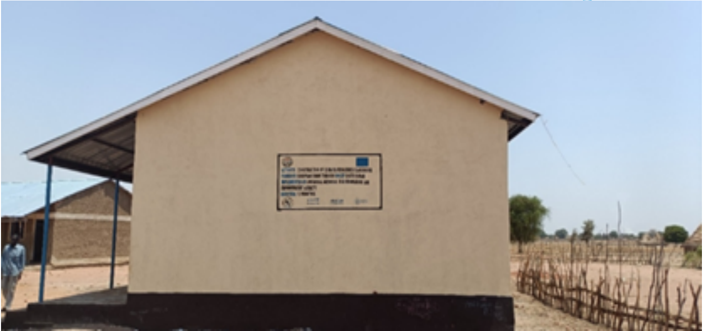
Side view of a Climate Resilience Classroom Block constructed by UNKEA in Majok Awan Primary School, Gogrial West County, Warrap State
