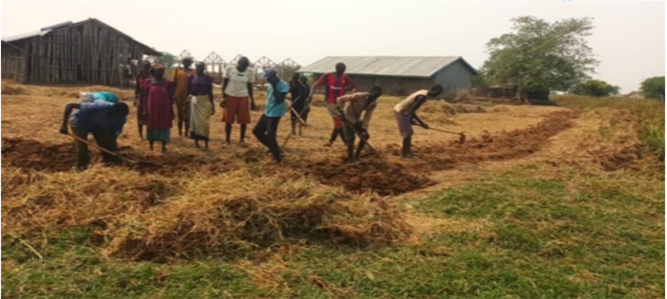
Dyke construction in Maker and Wechdeng primary schools by community members.
