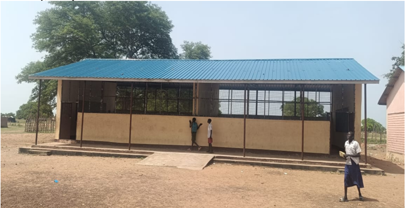
Front view of a Climate Resilience Classroom Block constructed by UNKEA in Majok Awan Primary School, Gogrial West County, Warrap State
