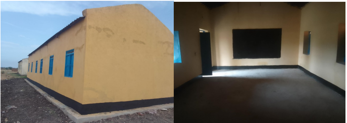
Rehabilitated classrooms in Nasir Secondary School in Nasir County, Upper Nile State
